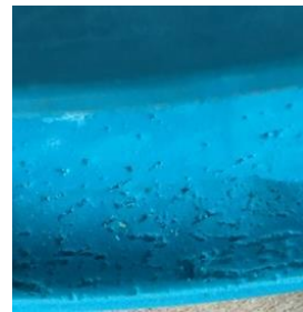
Uneven non-machined (cast) surfaces
