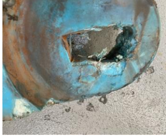
Deformation near the fixings
